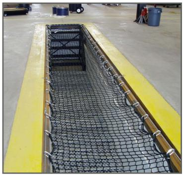
Add an enhanced level of safety to any vehicle service facility by protecting personnel from injury caused by accidental tripping, slipping or walking into an open pit. If your facility has service pits, you must comply with OSHA regulations by regularly using a protective covering or guard to prevent dangerous falls into the pit.
