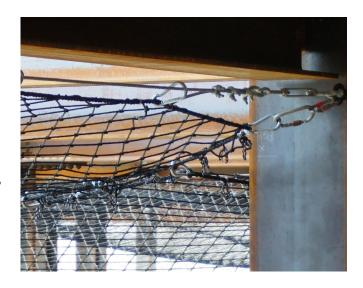
InCord's Steel Decking Netting Systems serve as a cutting-edge solution for enhancing safety measures at construction sites. These systems offer superior fall protection, easy installation, and versatile functionality.
