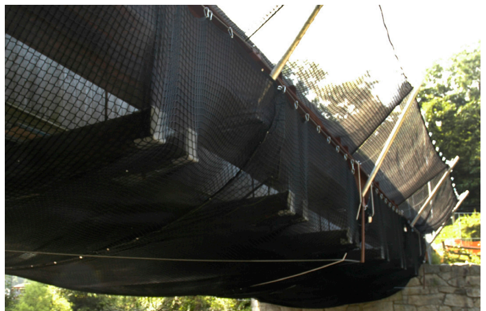
Combine PSN with RocBloc for complete containment.
